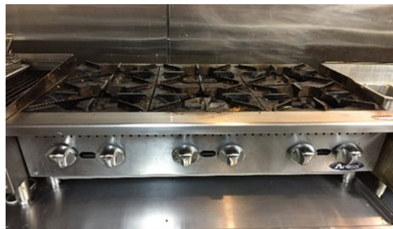
Equipment Elevated 4" Above Counter
